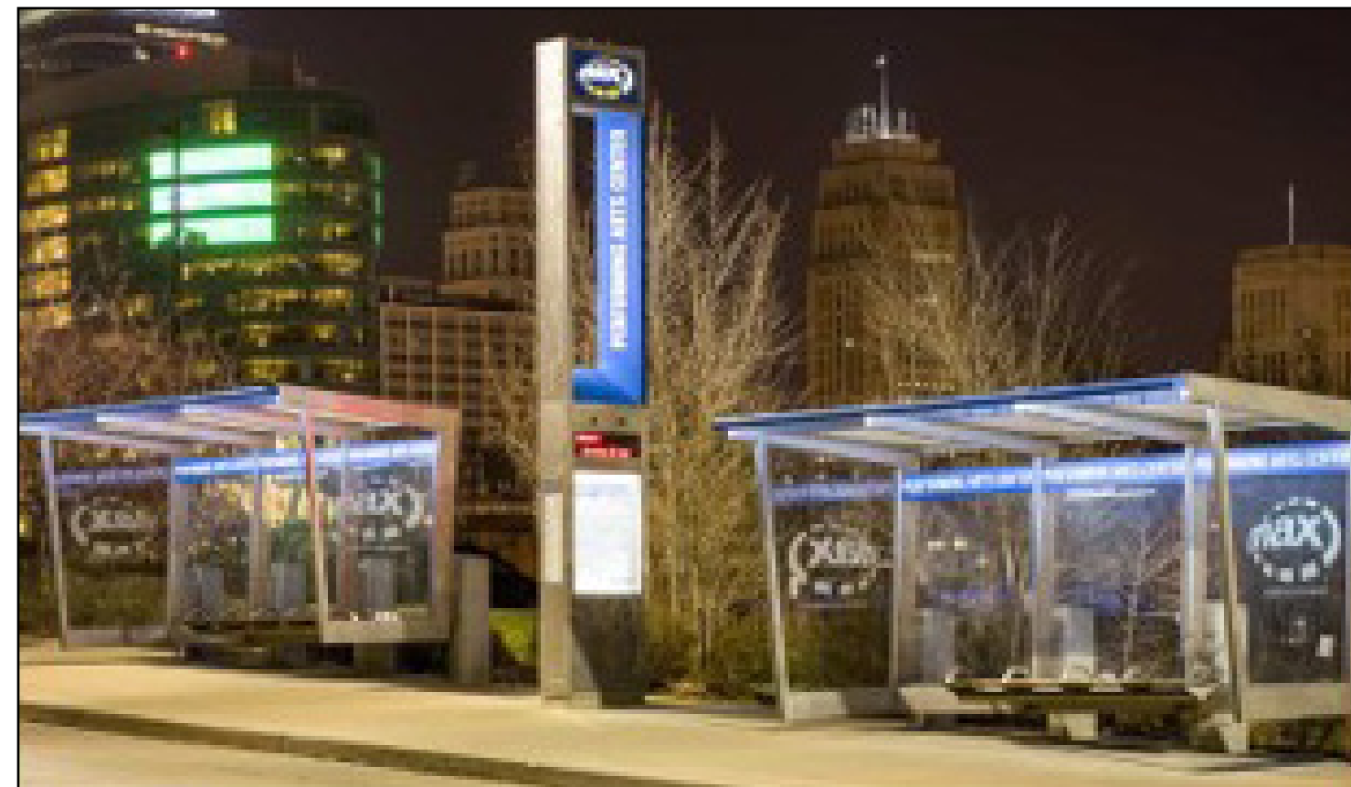
Stations with Lighting
